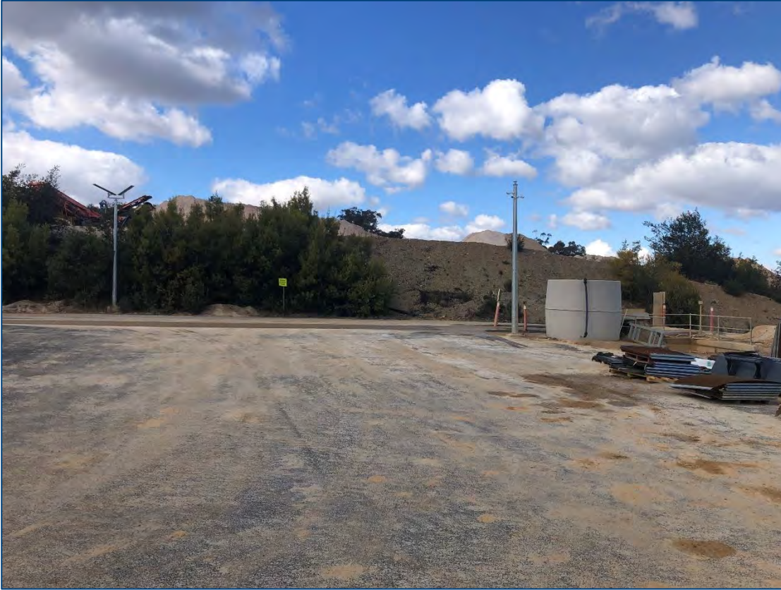
Photo 8.5 Processing Pad Haul Road Batter – Exposed Ground
