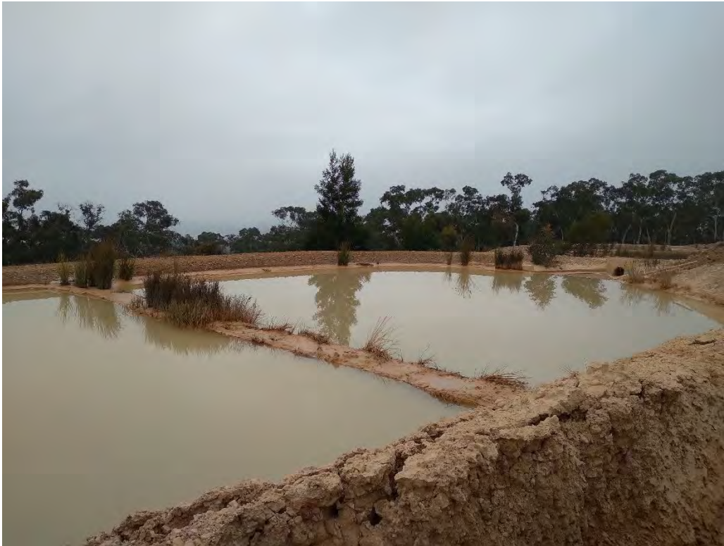
Plate 5 Silt settling cells below Wash Plant
