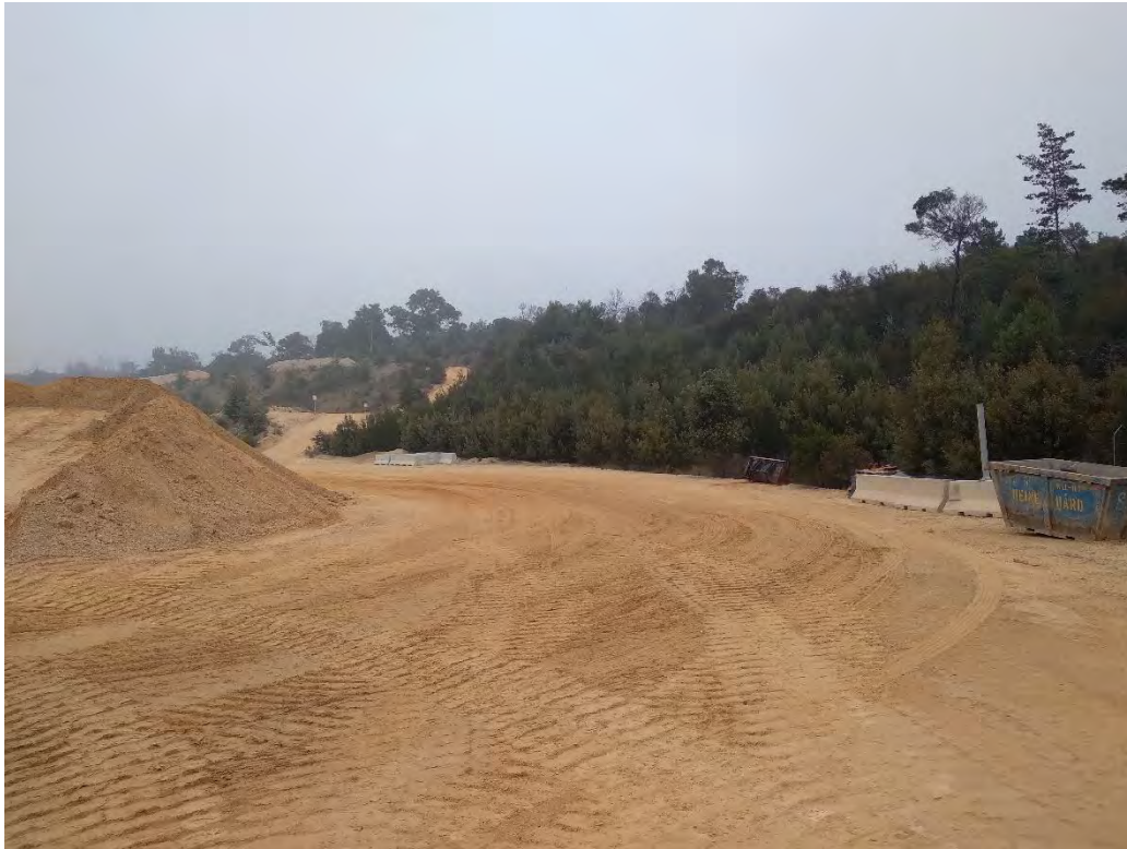
Plate 9 View from refueling area towards WSEA rehabilitation
