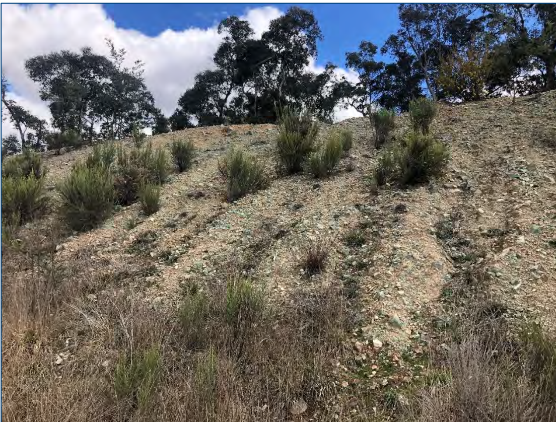
Photo 8.2 Western Stockpile Area Batter – Rilling and Exposed Ground 1
