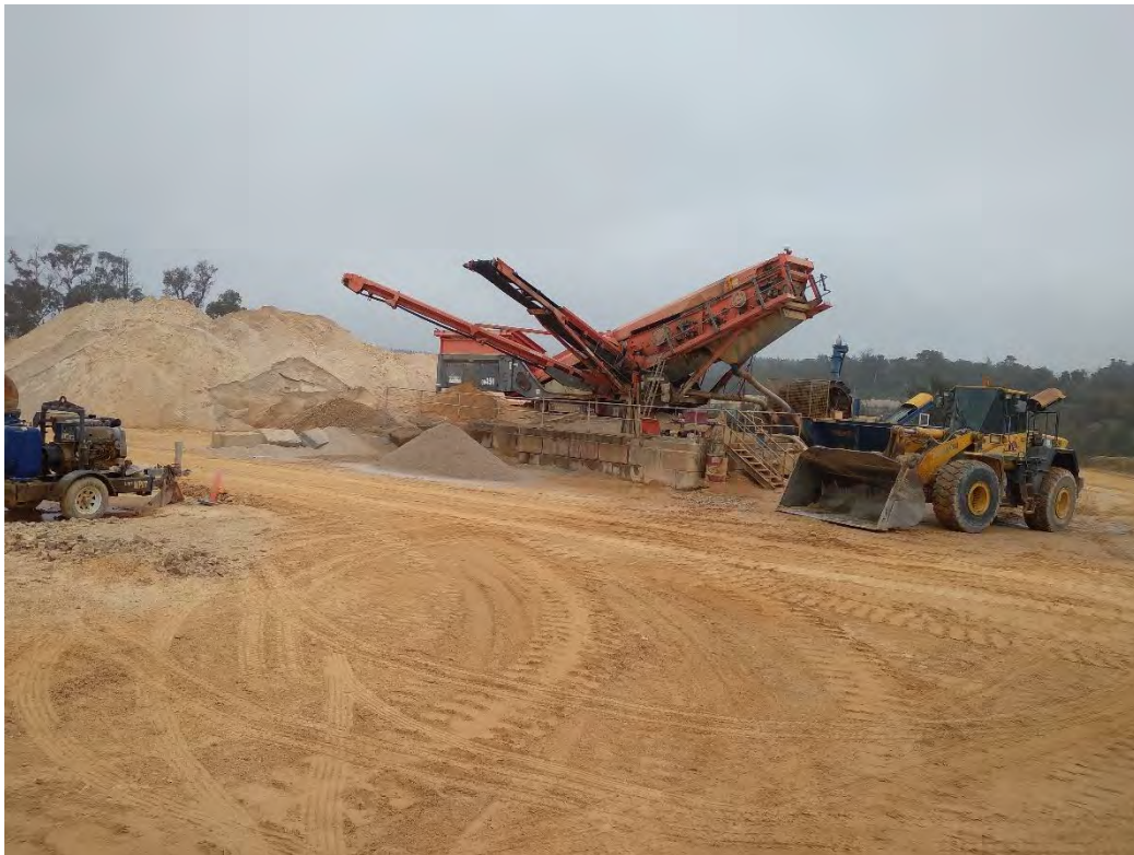
Plate 1 Wash Plant & loading area
