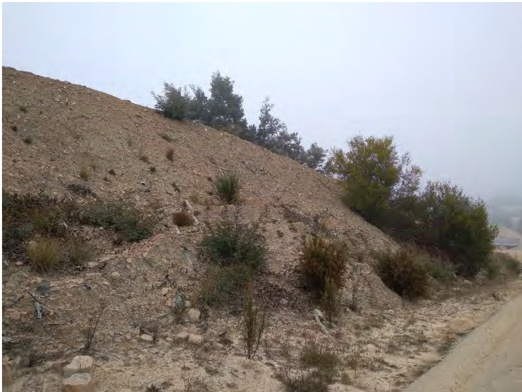
Plate 10 Bund adjacent site access road requiring rehabilitation cover
