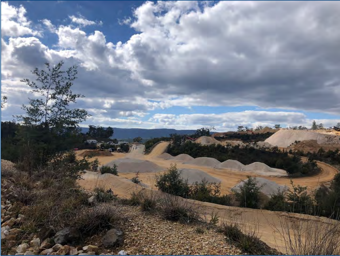
Photo 4.7 Main Stockpile Area
