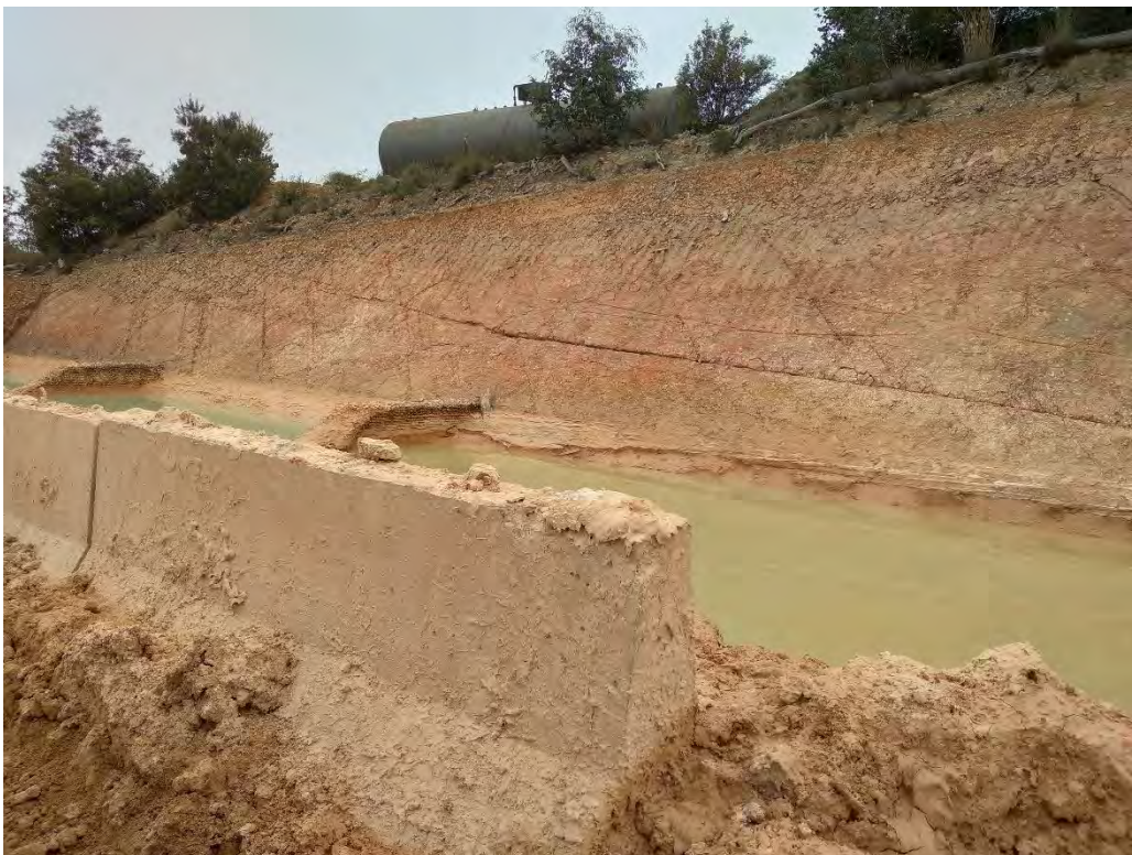
Plate 6 Settling cells adjacent Wash Plant area
