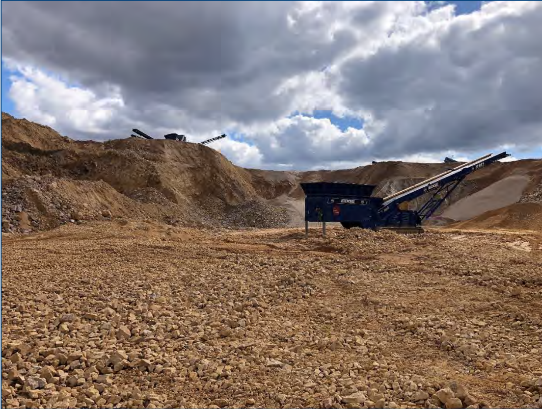
Photo 4.6 Road Base Crushing Unit
