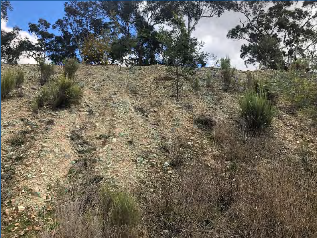
Photo 8.3 Western Stockpile Area Batter – Rilling and Exposed Ground 2
