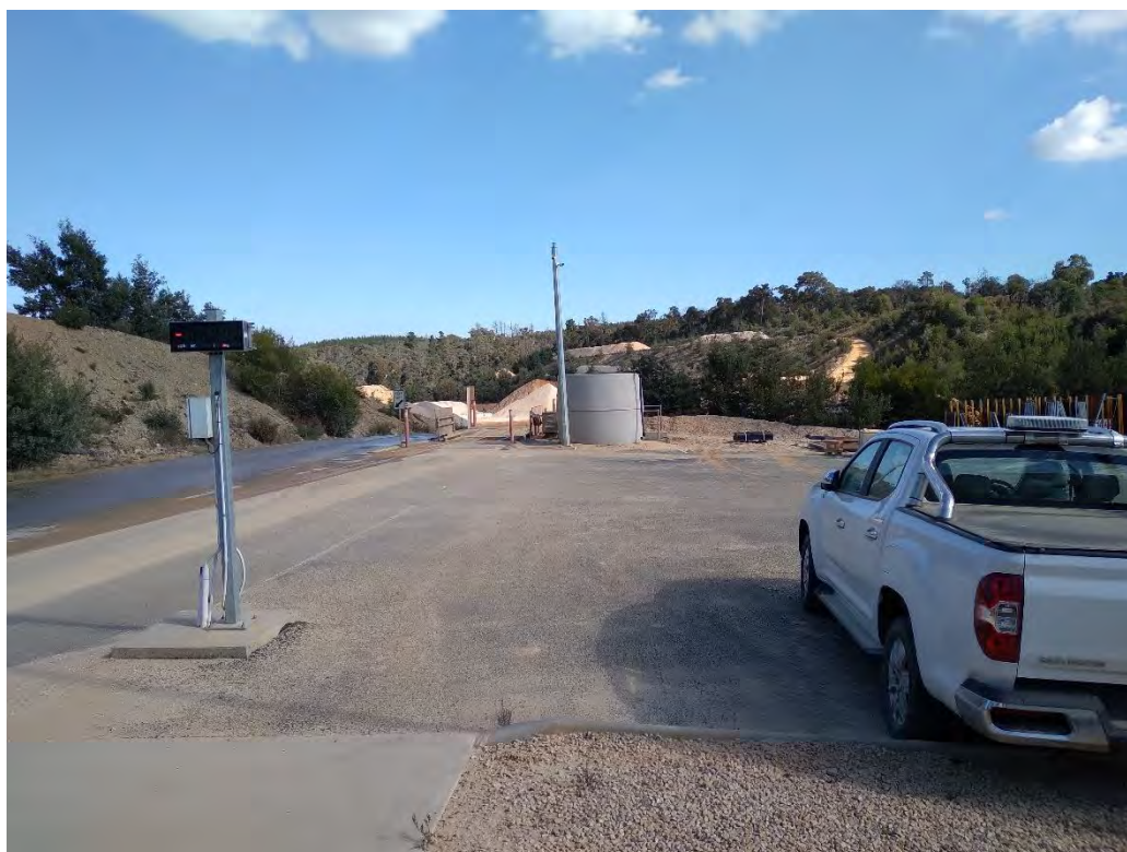
Plate 19 View from WQ site office toward wheel wash for trucks leaving site
