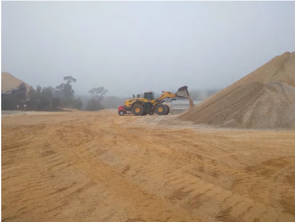
Plate 3 Product loading at Main Stockpile Area
