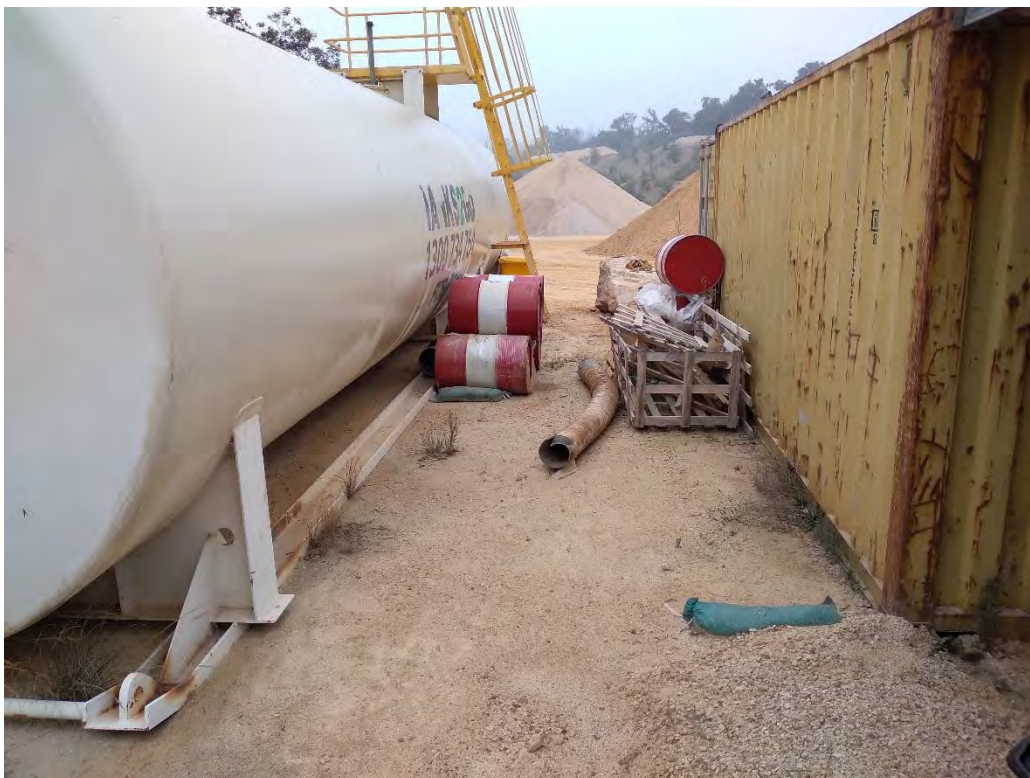
Plate 14 Oil drums located outside of bunded pallet
