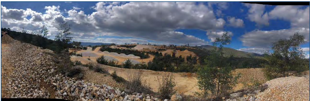
Photo 8.1 Panoramic View of the Quarry Site Identifying Retain and Re-established Vegetation
