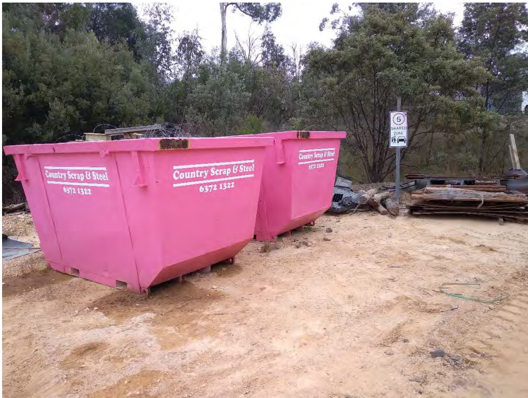
Plate 13 Example of segregated waste bins located on site
