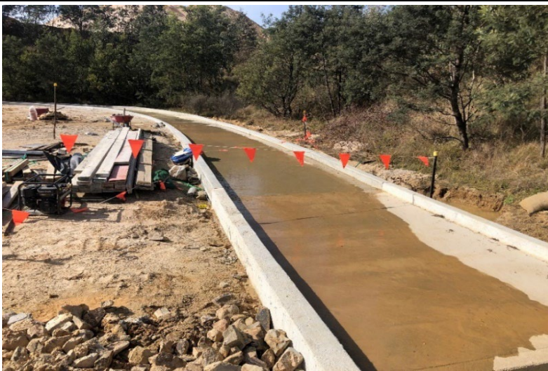
Photo 4.5 Concrete Drain Construction
