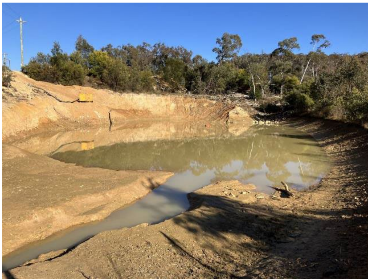
Photo 7.1 SB2 was observed to hold water at the July inspection, but the nominated storage capacity was maintained in compliance with the SWMP
