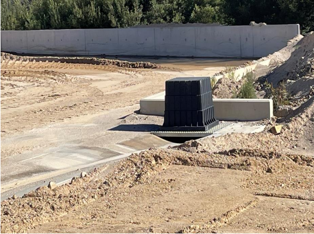
Plate 9 Water drain constructed around Sand Wash Plant
