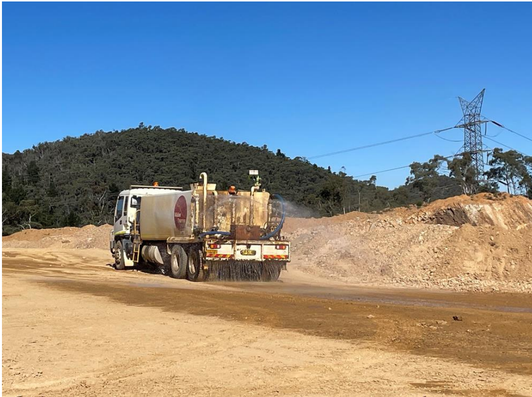
Plate 1 Water cart in use for dust suppression
