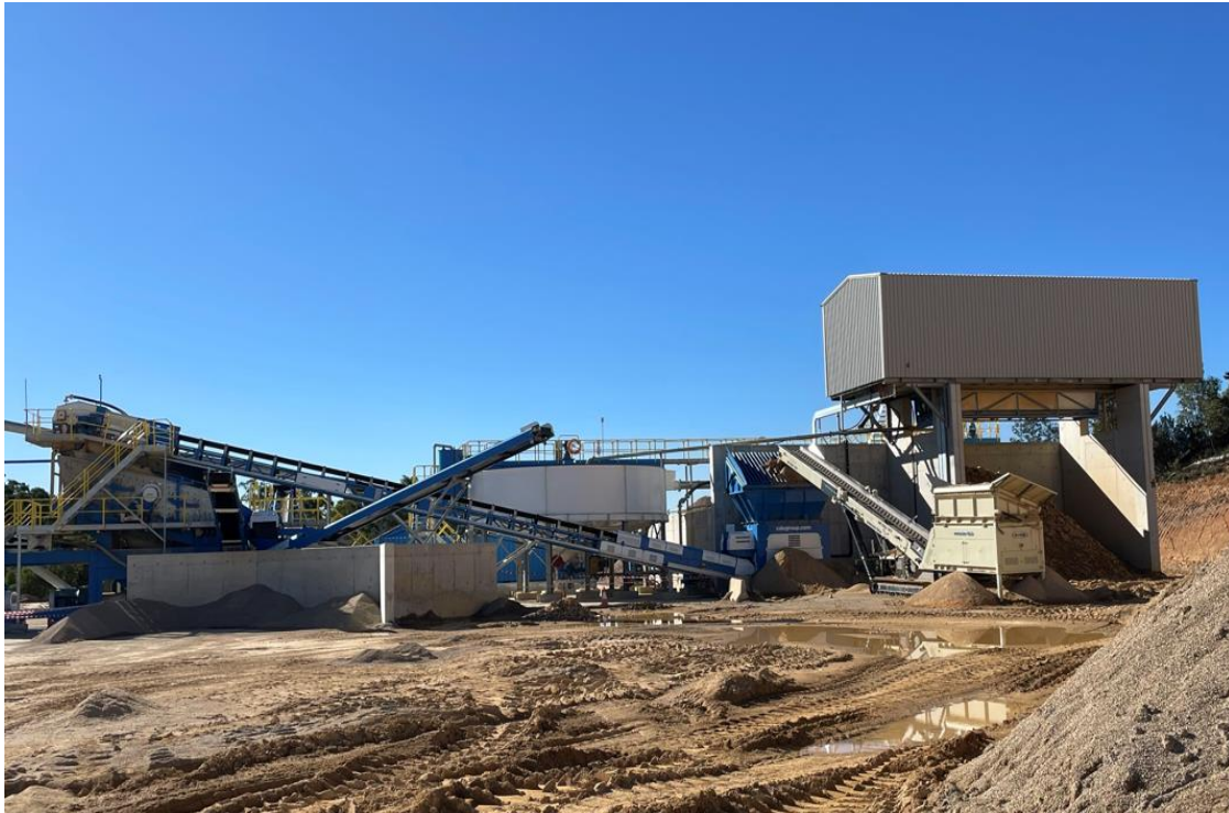
Plate 13 Sand Wash Plant constructed on site during the audit period
