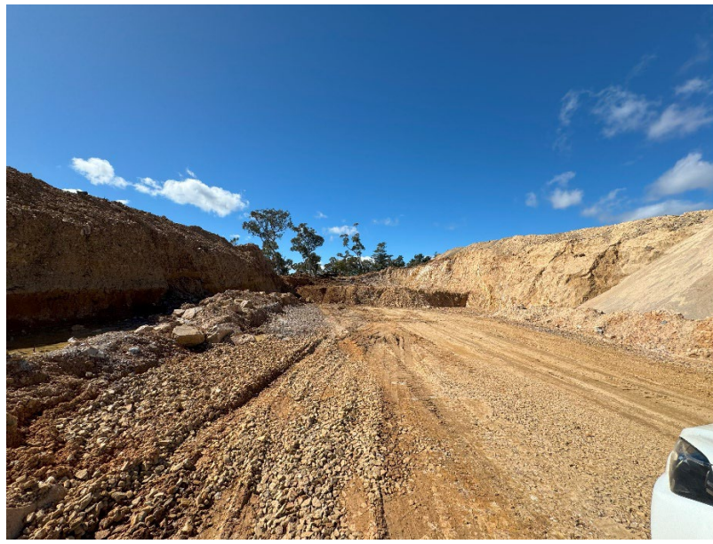
Photo 4-3 Extraction of previously stockpiled low value quartzite
