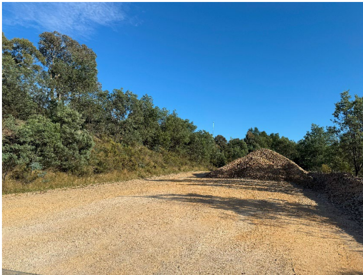
Photo 6-2 Revegetation of the Upper Batter of the Western Stockpile Area
